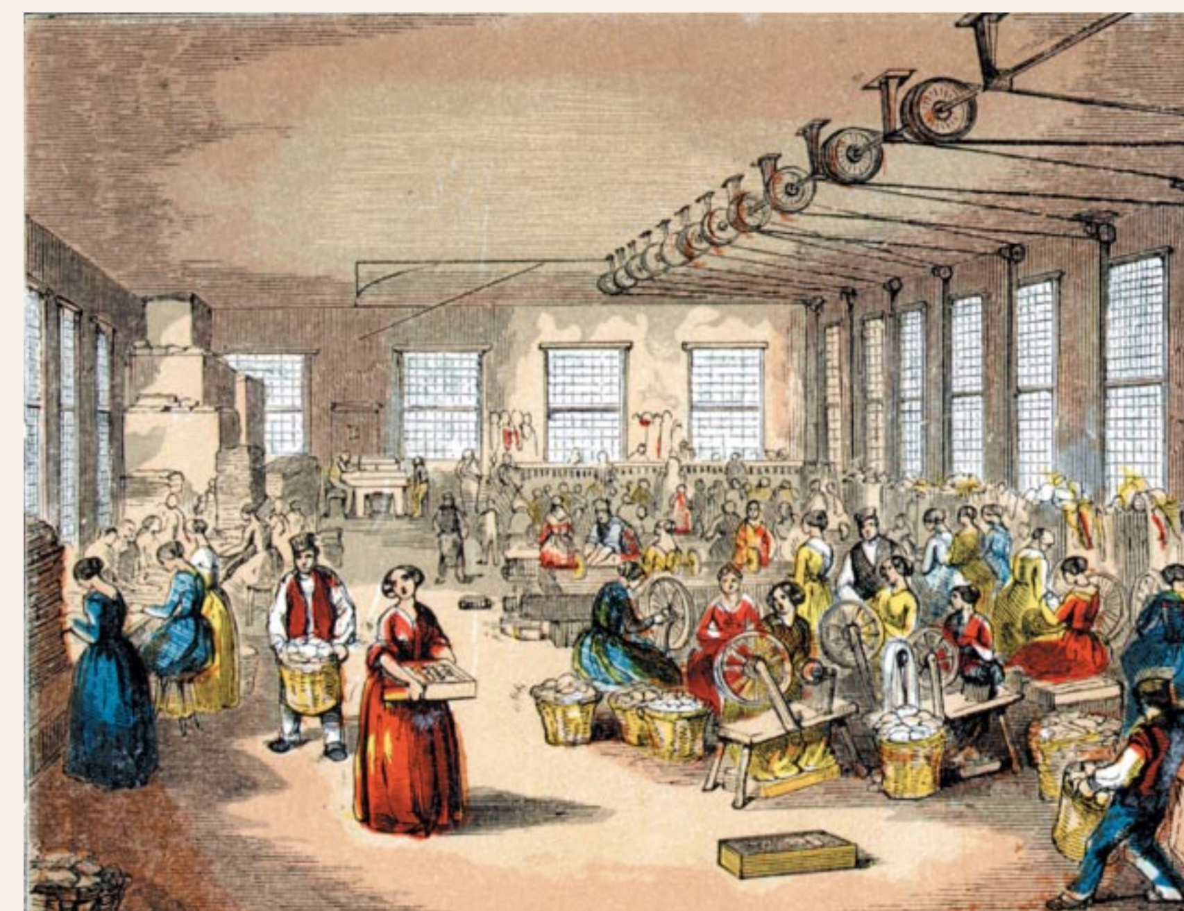
h Final winding, preparation and packaging of finished product.
