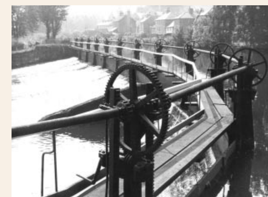
f The weir across the River Derwent in 1955 showing the sluice gate control wheels. These were destroyed by flooding about 10 years later.
